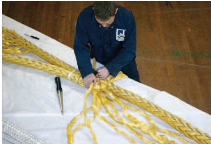
500 ton MBL sling at early stage construction.
